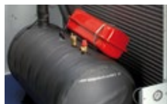
Built-in pumping module with or without storage tank.
